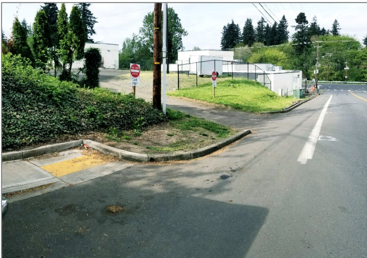
End of sidewalk NE 104th Street – Looking west to Hwy 99
